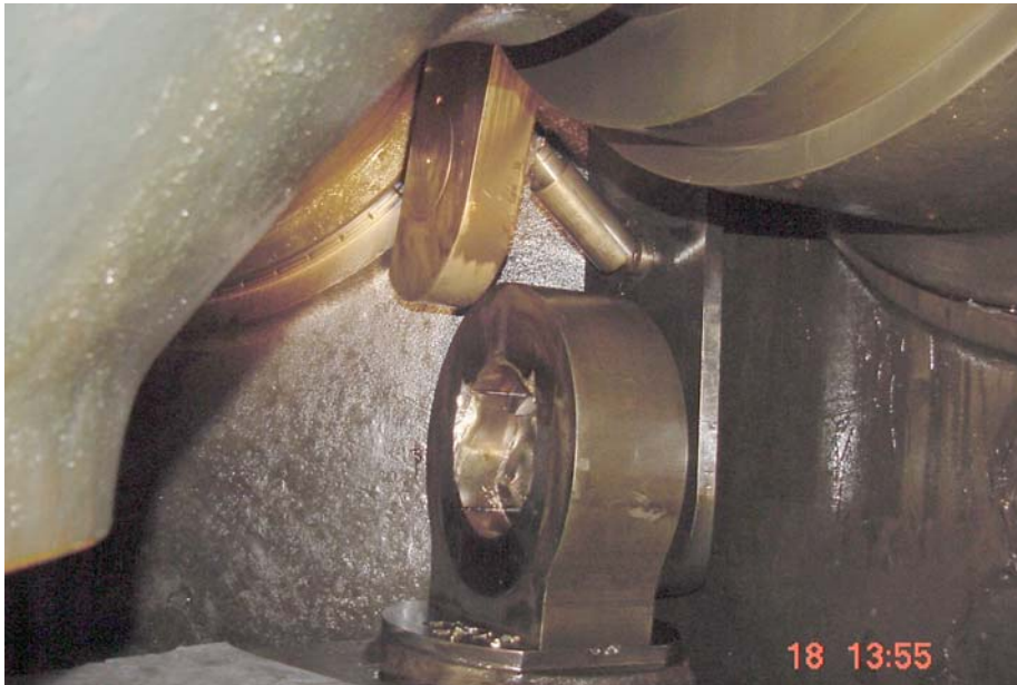
Photo A-2. Broken Linkage for Blade D, Lower Monumental Unit 1
